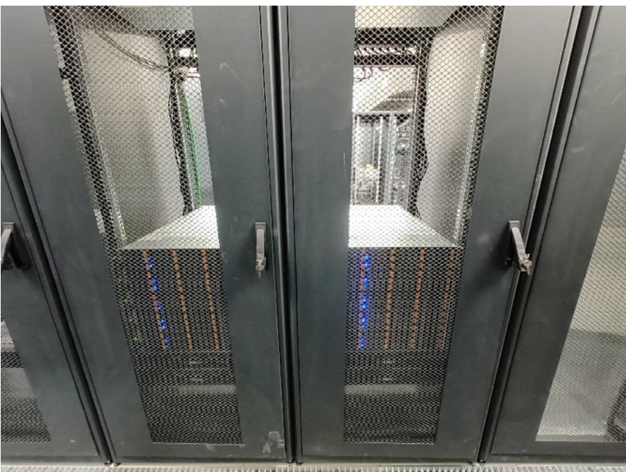
No. 1 rack cabinet hosting 9 multicore, high-memory and high-capacity servers.
